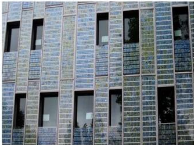
A building with facade covered by solar cells in Paris. (Photo Credit: La Citta Vita via Flickr )
