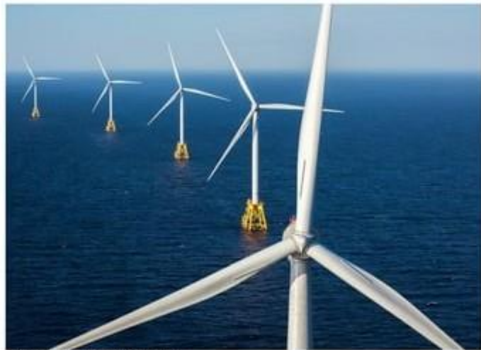
Photo of Block Island Wind Farm
