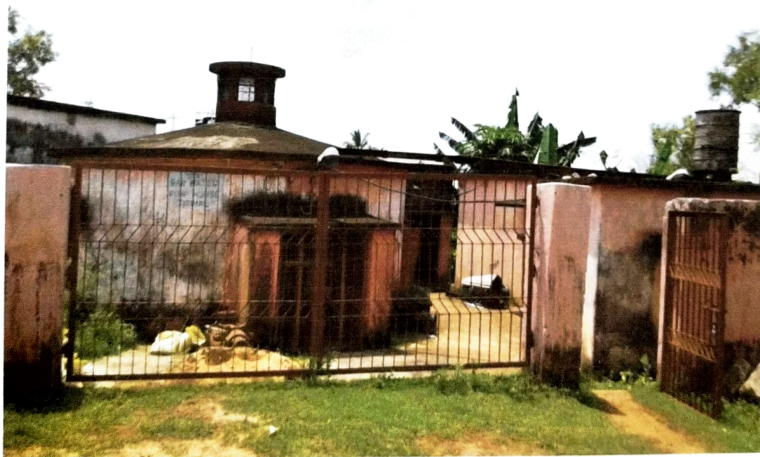
4. Water Pump House
