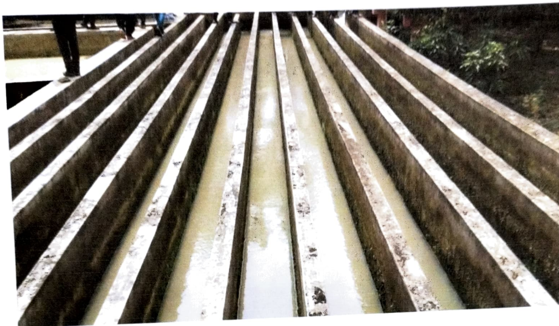
2. Baffle Wall at Treatment Plant
