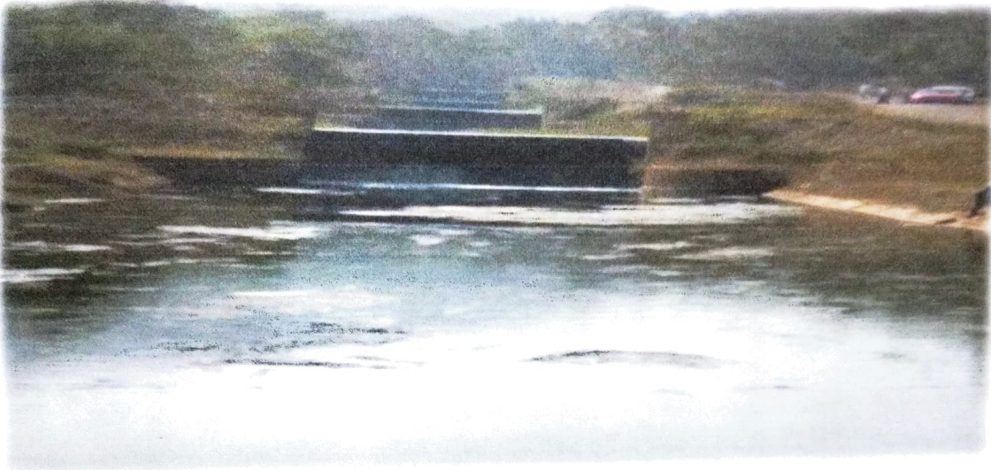
(Fig: -5, Stepped Canal Fall)
