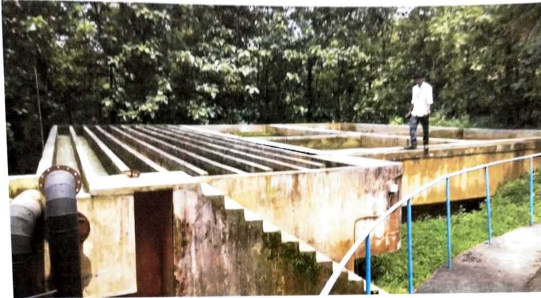
5. The Sedimentation Tank along with the Baffle Wall at Site
